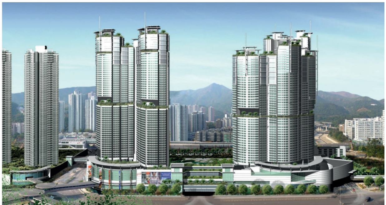
Hong Kong's mass transit rail system features oversite development above about half of its 87 stations, including Tai Wai station
