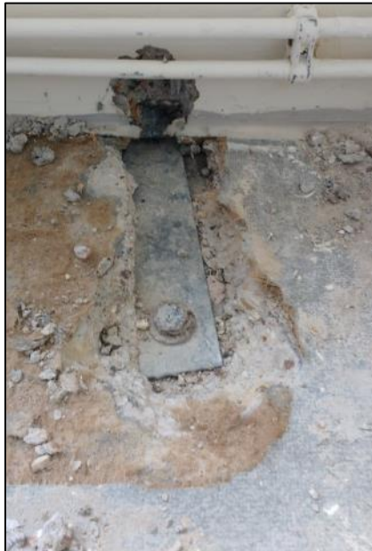
Figure 16 Non-structural wall panel to floor slab fixings exposed at locations 4 (LHS) and 5 (RHS). Chalk outline shows what the electromagnetic scanner located
