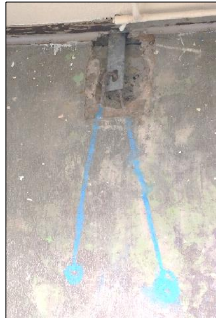
Figure 16 Non-structural wall panel to floor slab fixings exposed at locations 4 (LHS) and 5 (RHS). Chalk outline shows what the electromagnetic scanner located
