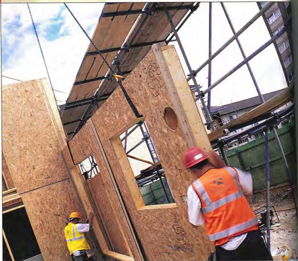
Kitchen wall panel with pre-cut hole for boiler flue.
