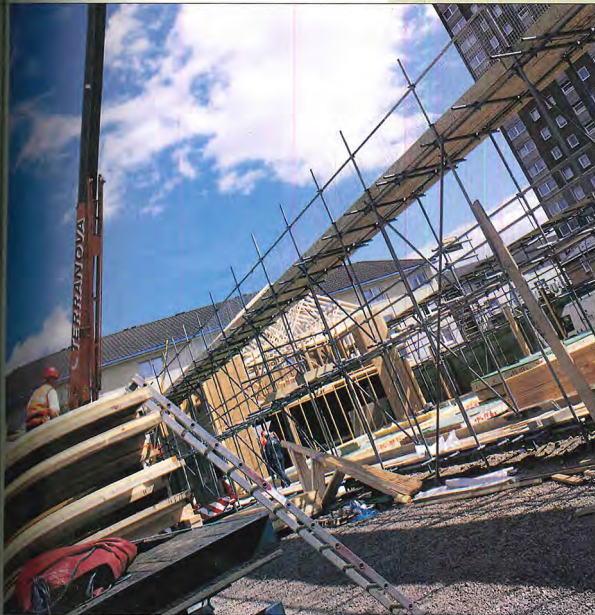
Components are unloaded directly into position.
