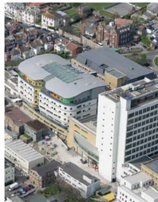
MEDICAL & HEALTH Royal Sussex County Hospital – (CAB) Clinical Administration Building £5,300,000
