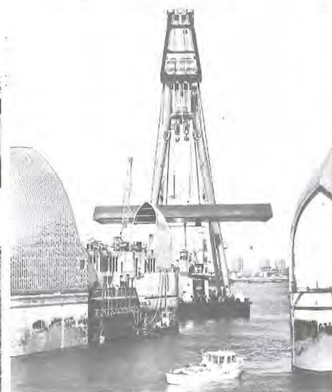
Below left: a giant Dutch barge crane being used to lower the steel rising sector gates into position.
