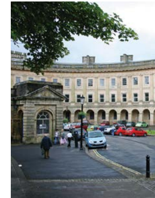
HOTEL, LEISURE & SPORT Buxton Crescent Hotel and Thermal Spa Phase 2 £35,000,000
