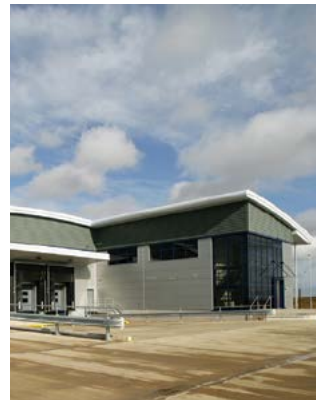
INDUSTRIAL Alwalton Hill, Peterborough – Plot 111 Warehouse £85,000,000
