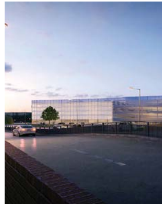
INFRASTRUCTURE Jaguar Land Rover – Multi Storey Car Park £30,000,000
