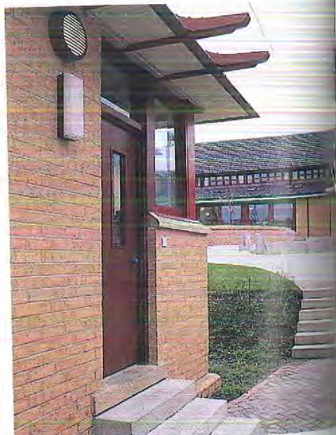
Above: Gutter and eaves allow no place to climb.
