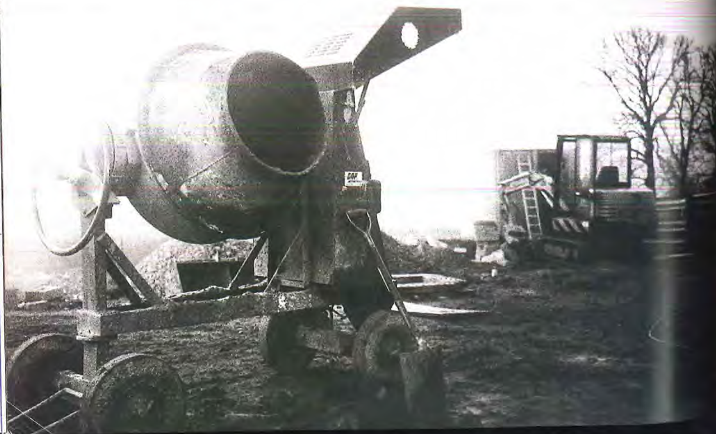
Below: Construction equipment stands idle in the Cumbrian countryside.
