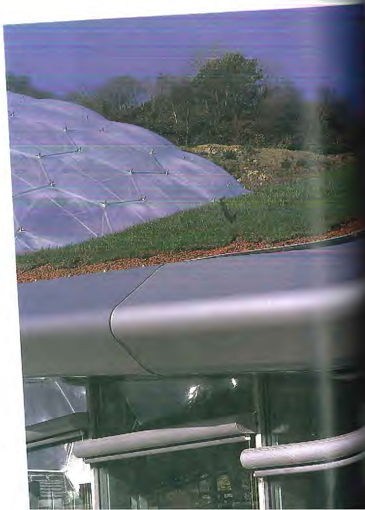
The biomes are connected by a restaurant topped by a turf roof.
