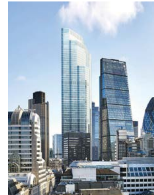
COMMERCIAL & RETAIL 22-24 Bishopsgate – Office/Retail/Restaurant £500,000,000
