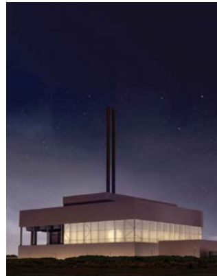
INFRASTRUCTURE Beddington – 26MW Energy Recovery Facility £20,000,000
