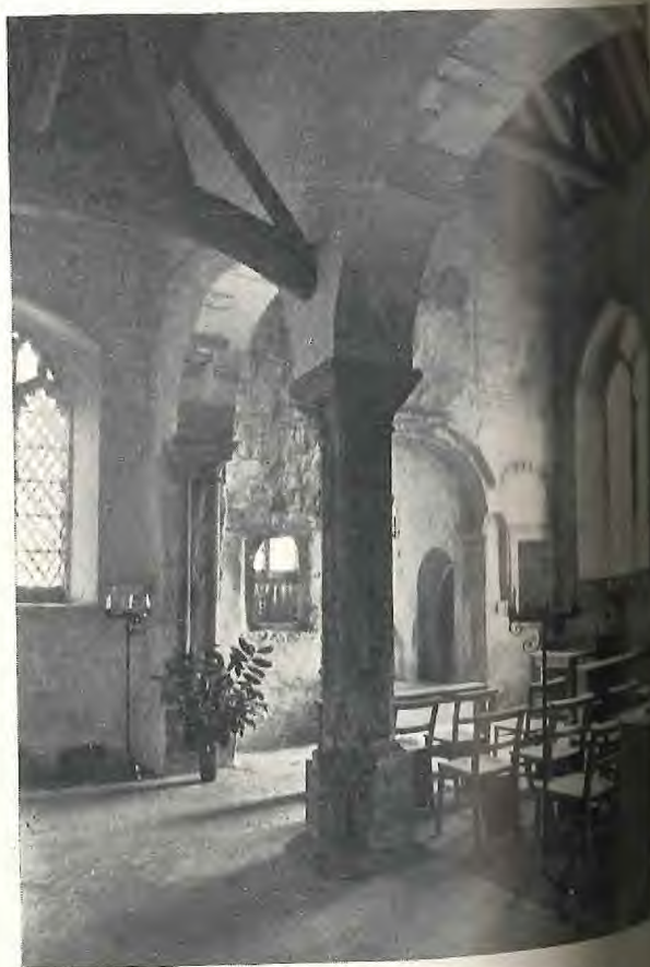
NORTH AISLE (LOOKING EAST) AFTER RESTORATION.
