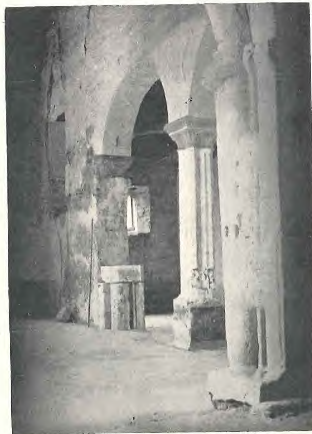
NORTH AISLE (LOOKING WEST) BEFORE RESTORATION.
