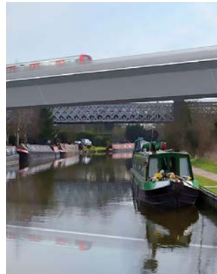
INFRASTRUCTURE Croxley Rail Link Project £70,500,000
