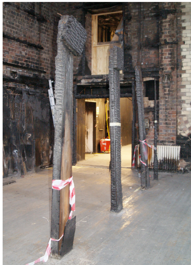
1. Timber post post-fire 2. Upper post. 3. Upper post comprised of two composed. 4. Timber plate covering joints junction. 5. Plan of the post and timber plate. Thick nails fixing lower and upper post highlighted in circle.
