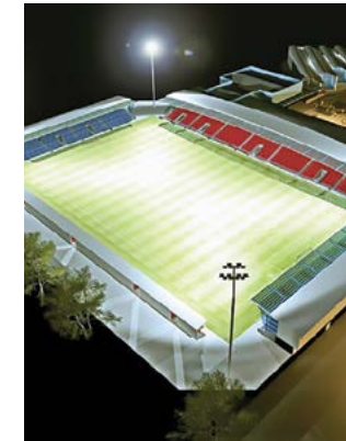
HOTEL, LEISURE & SPORT York Community Stadium £37,000,000
