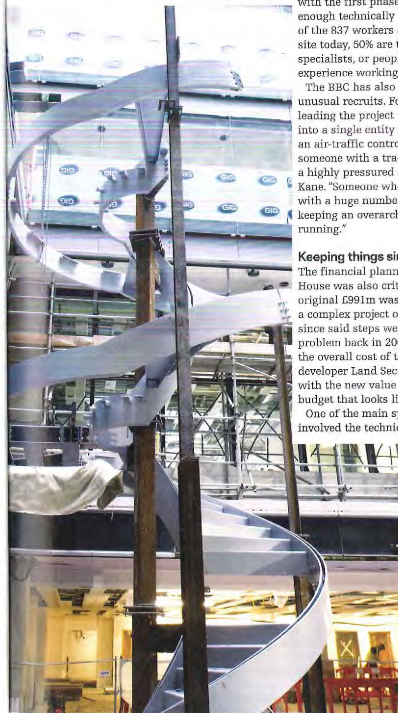
Far left: The floors of the extension have been built around a 43m-high atrium
