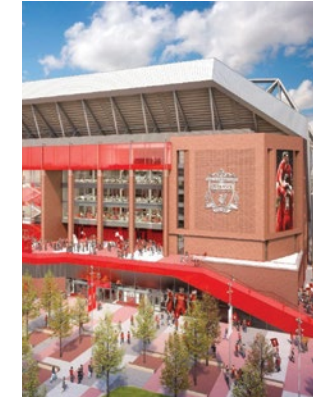
HOTEL, LEISURE & SPORT Liverpool Football Club – Anfield Stadium Expansion – Main Stand – Phase 1 £75,000,000
