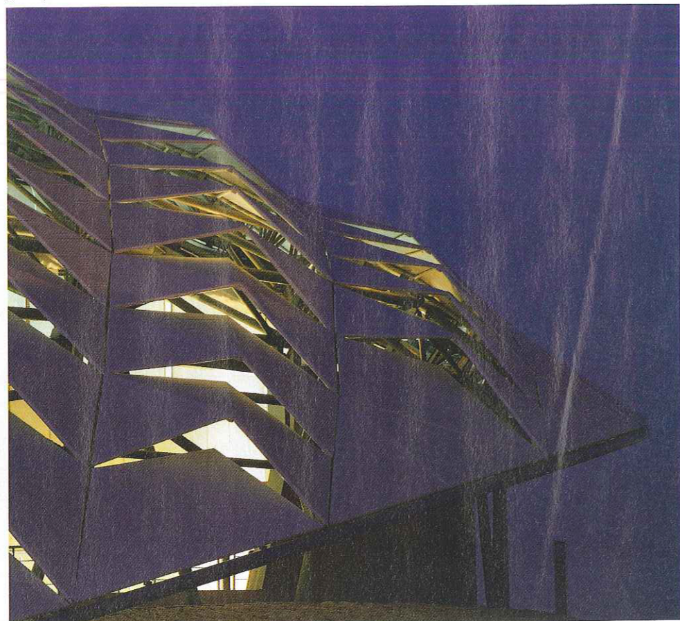
The PVC roof panels create north facing "cowls" that block out direct sunlight but allow a degree of natural light onto the grass pitch.
