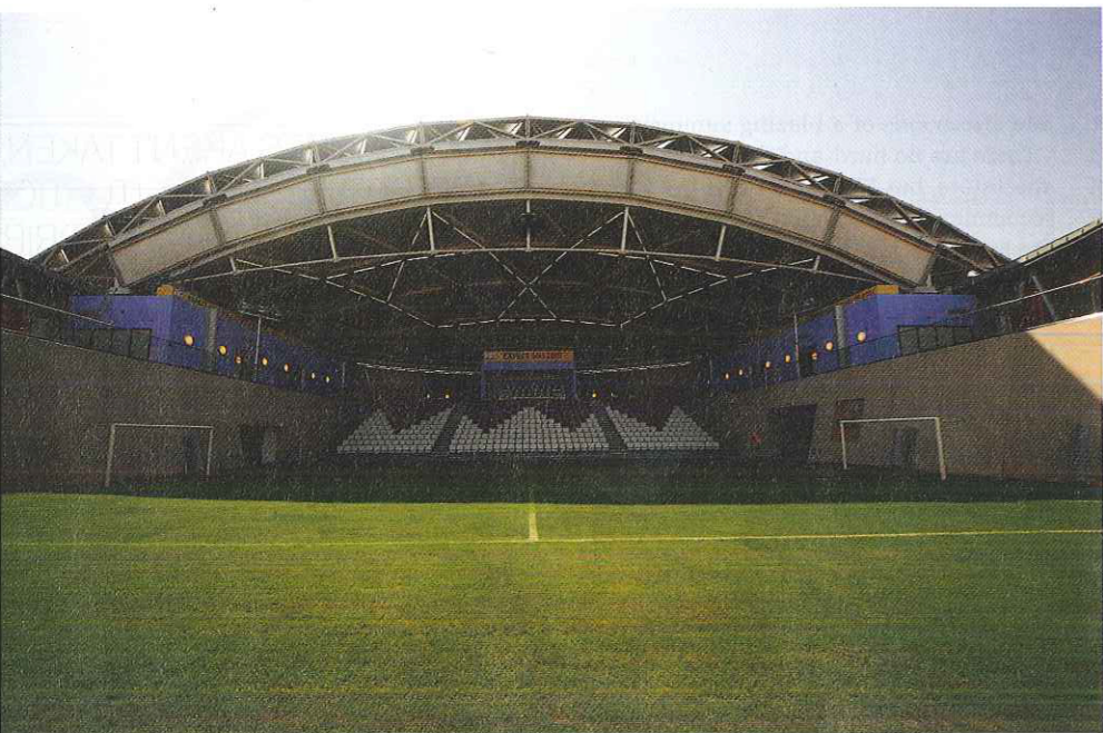
World Cup matches cannot be played under cover, so a rotating roof protects the showcase from the sun and wind, but opens the pitch to the sky when needed
