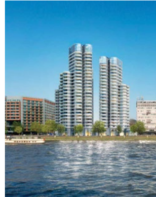
RESIDENTIAL The Corniche – Hampton House Redevelopment – Nine Elms £73,400,000
