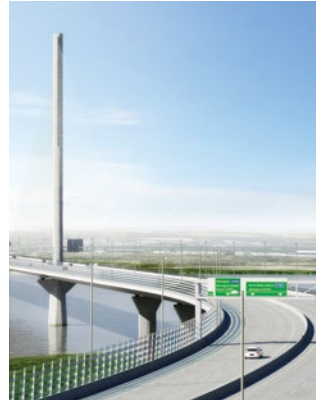
INFRASTRUCTURE Mersey Gateway Bridge – Highway Improvement Works £37,000,000
