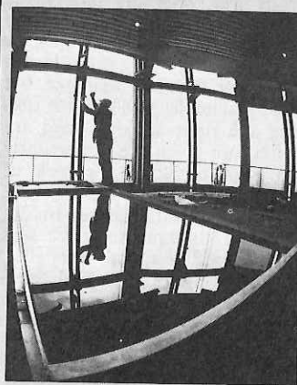
"Reflection": preparing window frames prior to installation.
