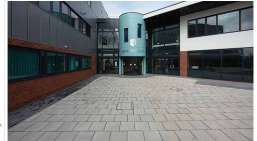
Below: Whitmore Park was delivered by the same team as Campsmount Technology College - which was also built to standardised design; Bottom: Nursery and reception areas at Whitmore Park flow between internal and external space
