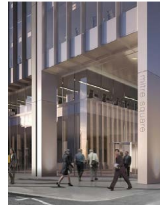
COMMERCIAL & RETAIL Creechurch Place Development £95,000,000
