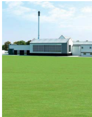
INDUSTRIAL Teaninch Distillery – Project Brae £50,000,000
