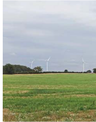
INFRASTRUCTURE Jacks Lane Wind Farm £21,000,000
