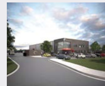
Aberdeen Energy Park Expansion
