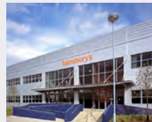
Dirft II Expansion Zone 3 – Sainsburys Distribution Centre
