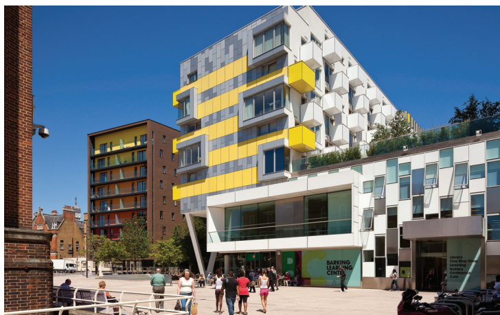
Triple-glazing is one emissions-saving solution for high-quality apartments such as these 515 mixed-tenure homes in Barking
