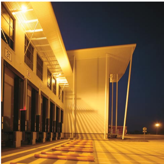
24 hour energy efficient intelligent lighting
