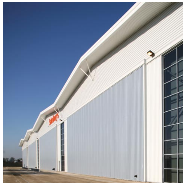
Insulated closed doors policy to prevent energy leakage
