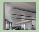
Radiant sails cooling with solar film to glass and energy efficient downlights
