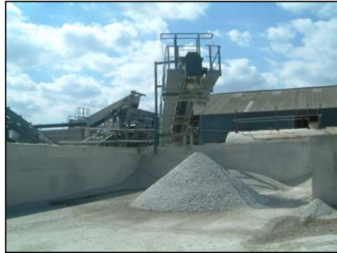
Day Aggregate's concrete crushing facility where Unilever House demolition concrete was reprocessed for reuse within the industry
