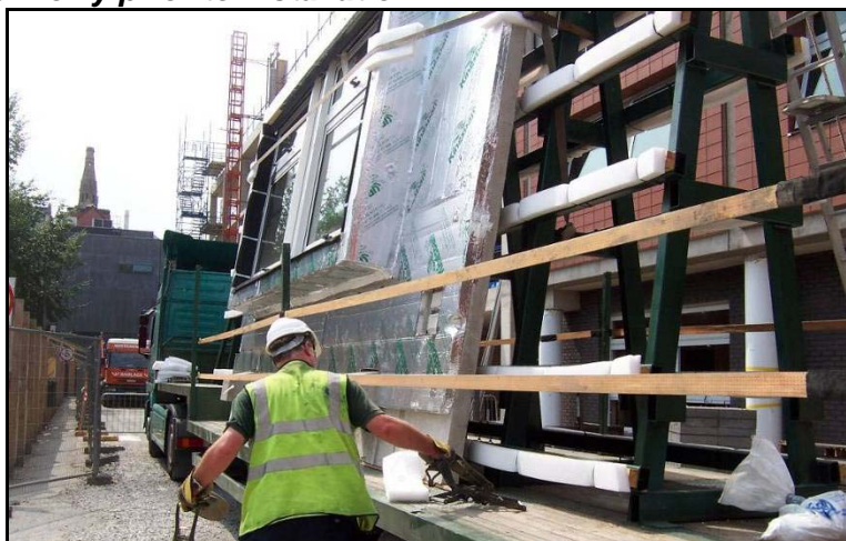
Figure 1 - Panel on lorry prior to installation
