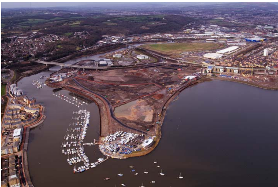
Site during reclamation project
